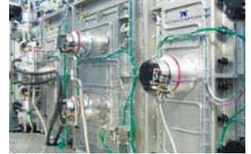
Systems for glass coating with HiPace turbopumps from Pfeiffer Vacuum for Leybold Optics GmbH
